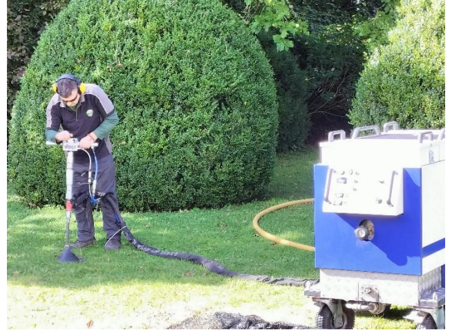
Matt Vaughan demonstrating the Geo Tree system.
