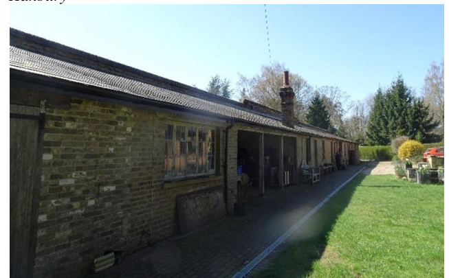
Service buildings for Marnock's kitchen garden at Hitcham House (Claire de Carle)
