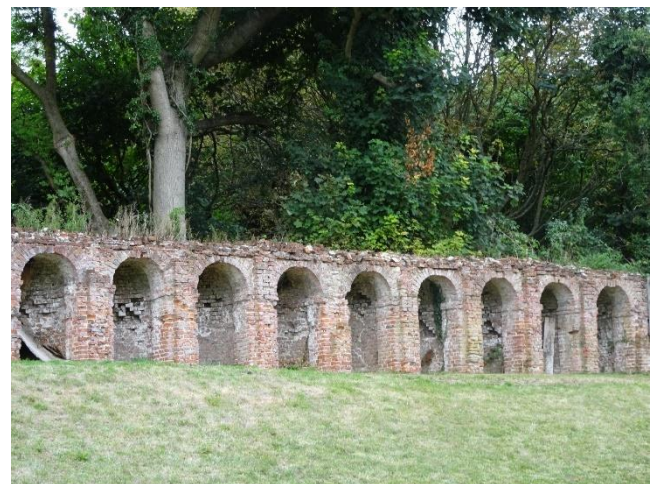
Raised terrace and arcaded wall in 2 nd enclosure
