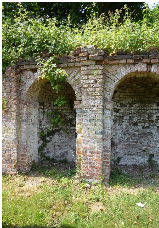
Two arches in wall in detail– use not identified G Huntingford
