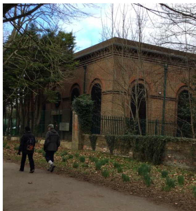
Pumping station, south facade
