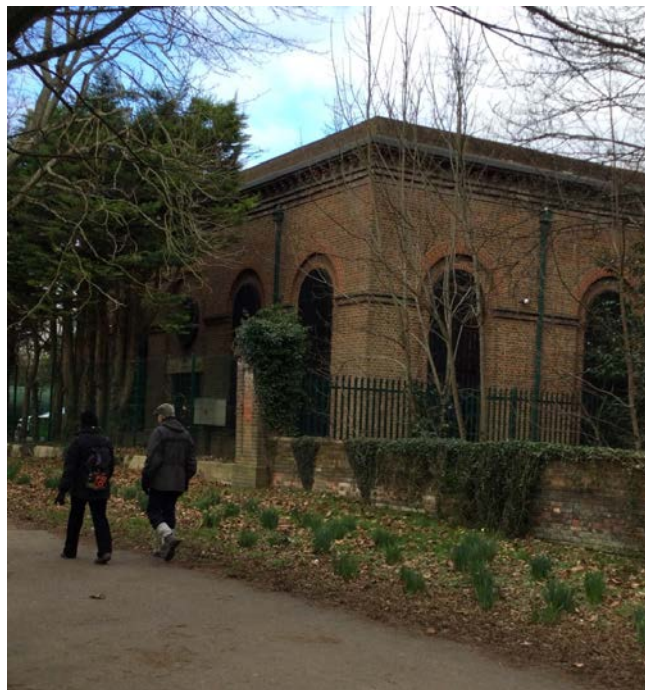
Pumping station, south facade
