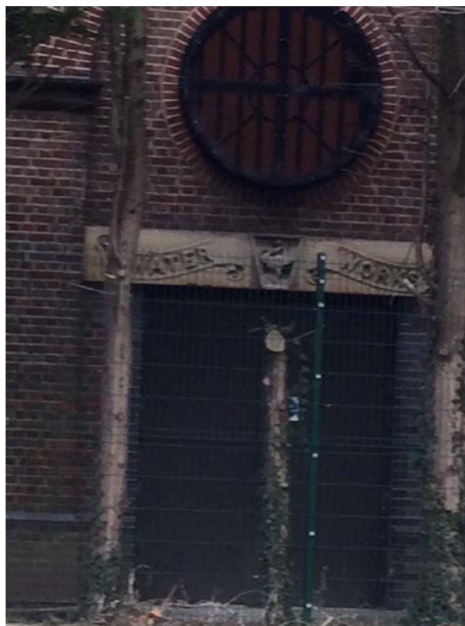
Former entrance to the pumping station
