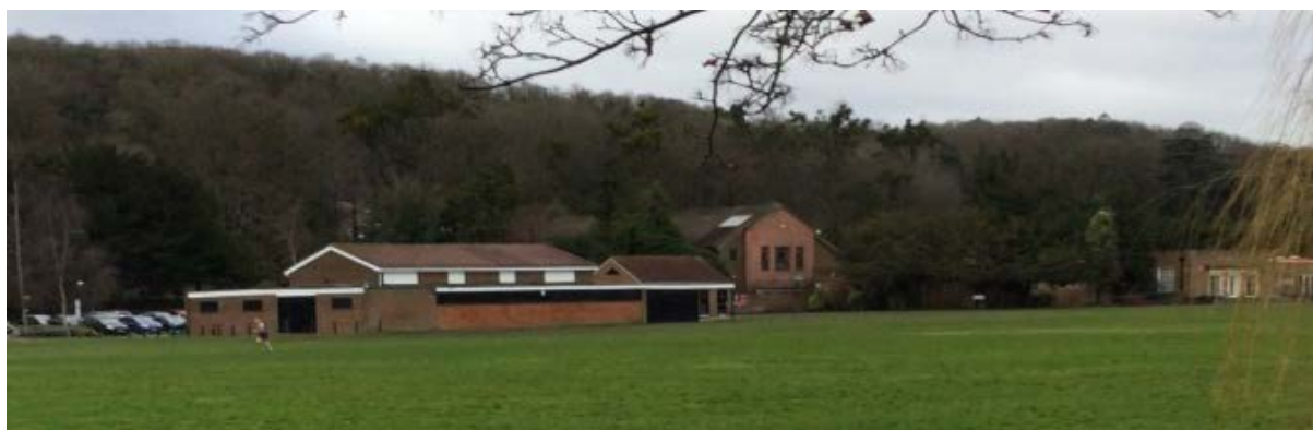
Changing rooms, public lavatories and Lido complex
