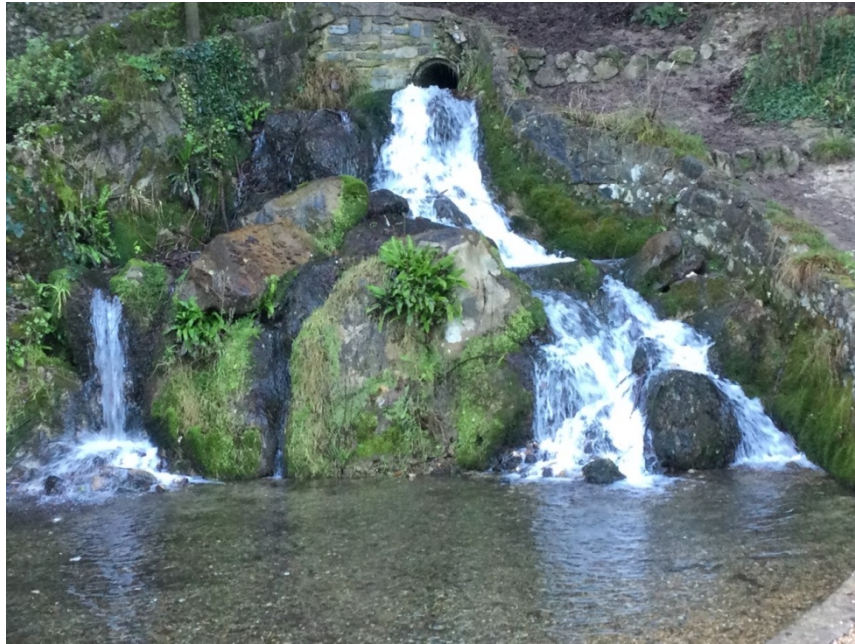
The Cascade at the SE end of The Dyke
