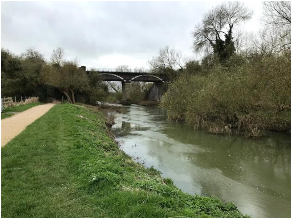
Iron Trunk Aqueduct
