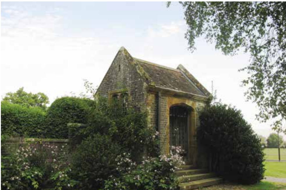
FIGURE 2 Akeley Wood: Ernest George's 1911/12 Tudor-style brick and ironstone gazebo as part of his Arts and Crafts style garden additions ( Ken Edwards )
