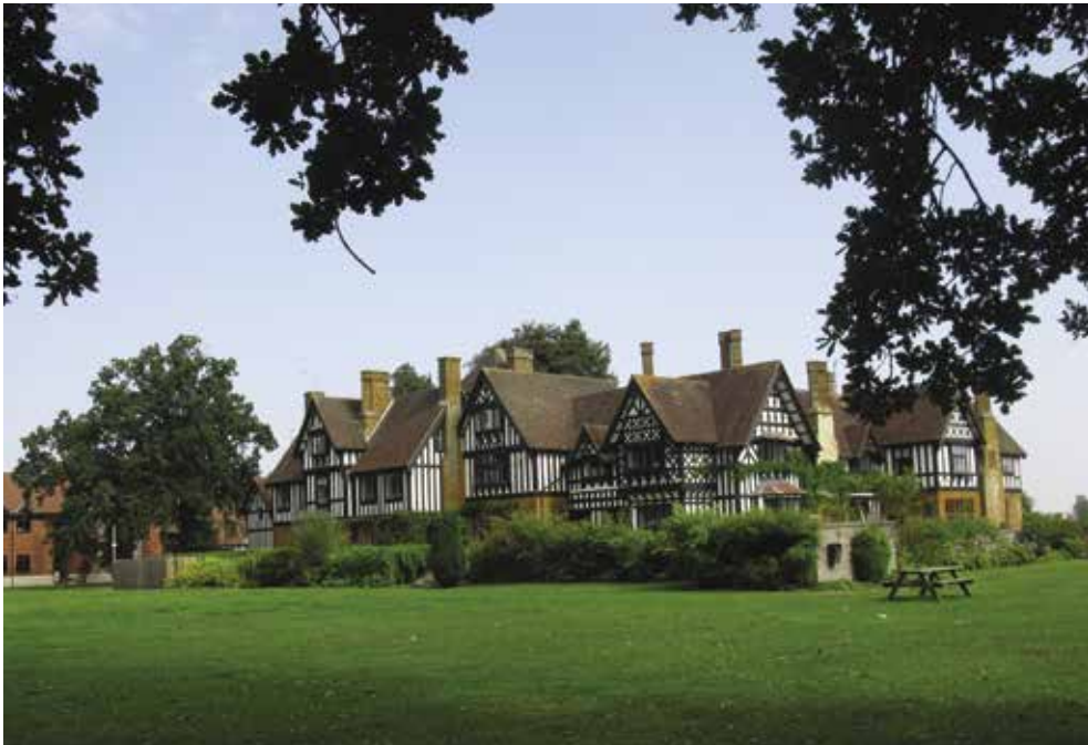
FIGURE 1 Akeley Wood: George Devey's first large-scale country house, 1860s ( Ken Edwards )
