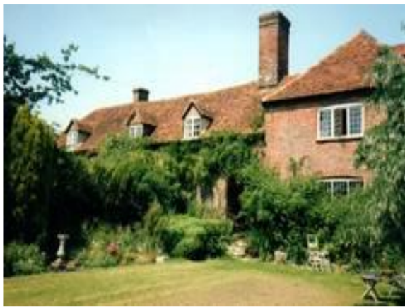
The farmhouse from its private garden to the south
