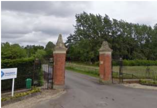
Grendon Underwood. The gate piers, main entrance (Google Earth)
