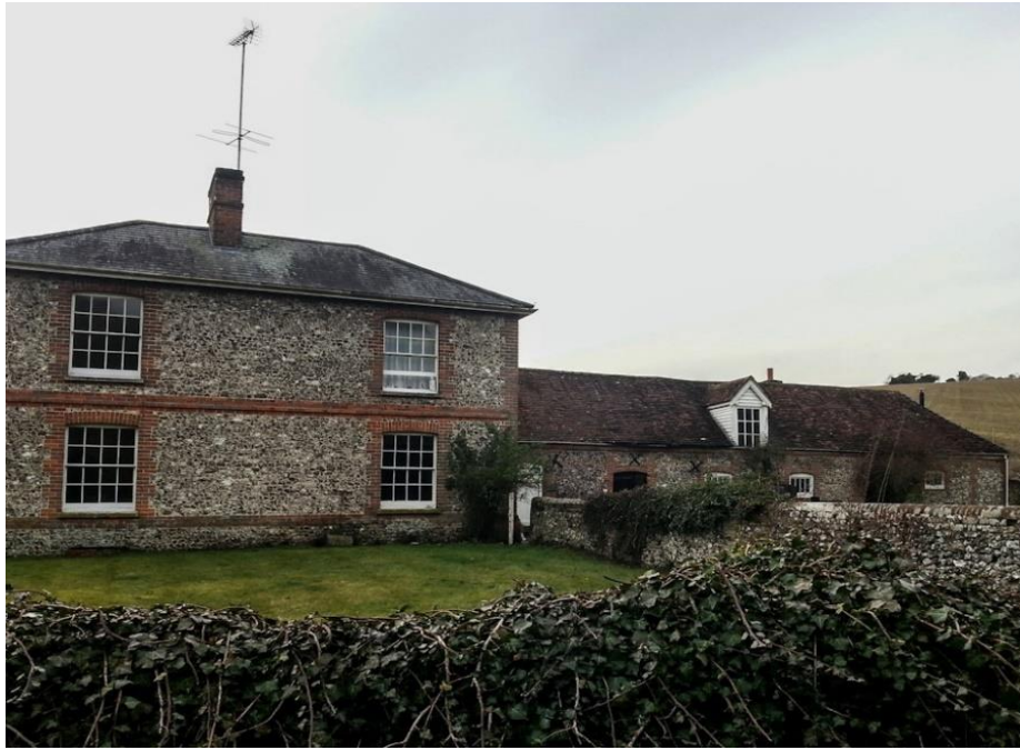
East front, 2019 (Photo: John O'Dwyer) The single-storey building, previously a cowshed, once served as a studio.
