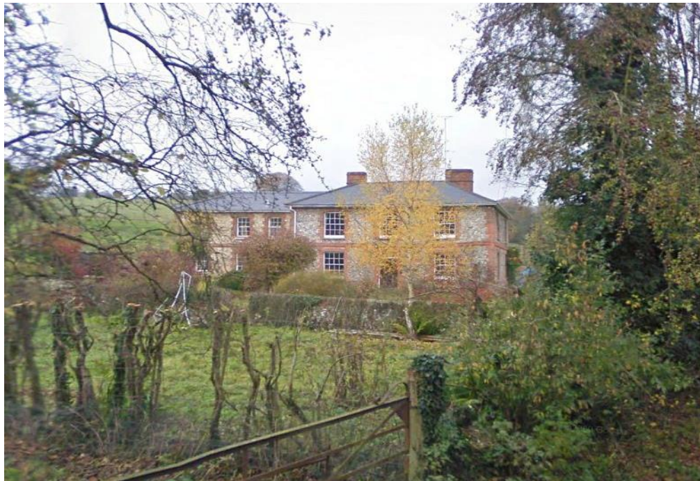
South front, 2018 (Photo: Google Earth)
