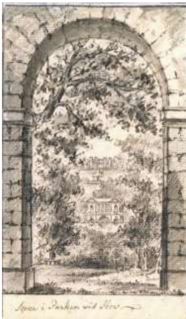
View through the Doric Arch F Piper
