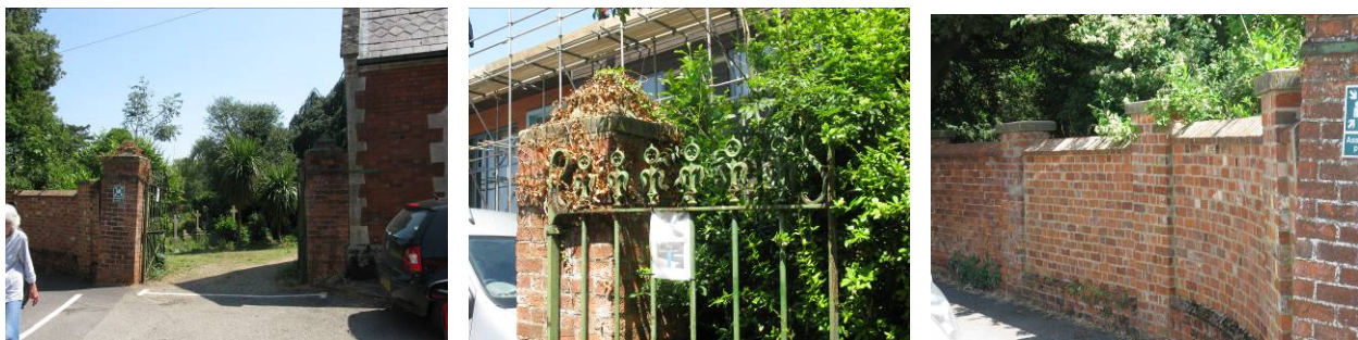
Gateway and boundary wall
