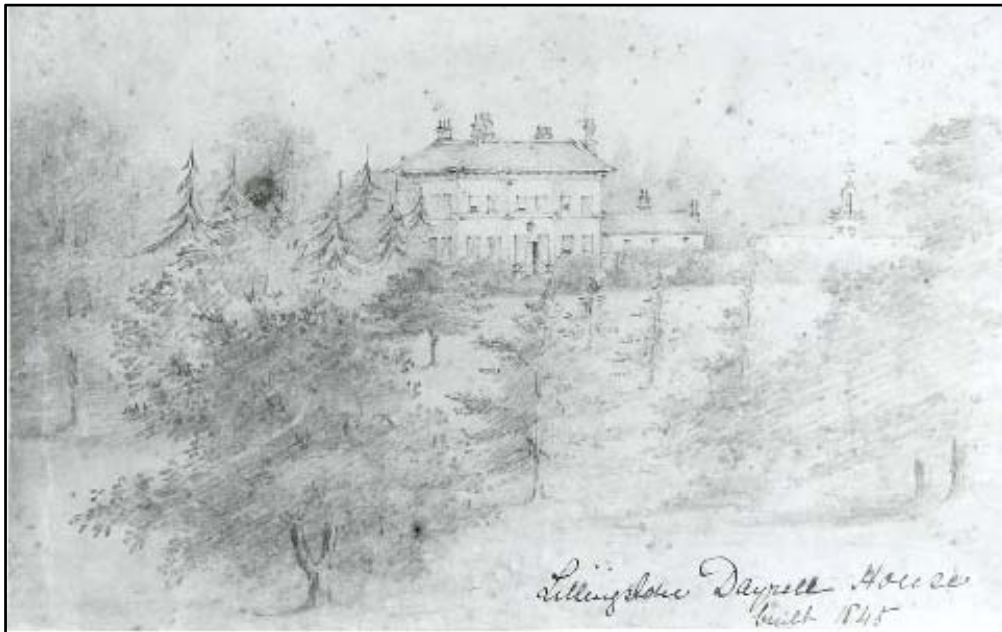
'Lillingstone Dayrell House built 1845' Historic England Archive
