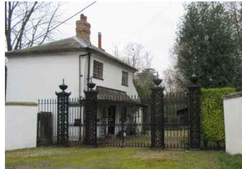
C19 Former entrance Lodge and
