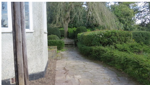
South Paved Terrace looking East
