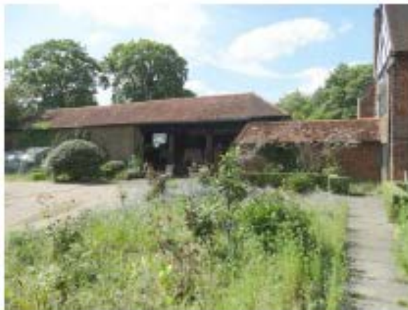
The single storey extension with the wooden Doric columns
