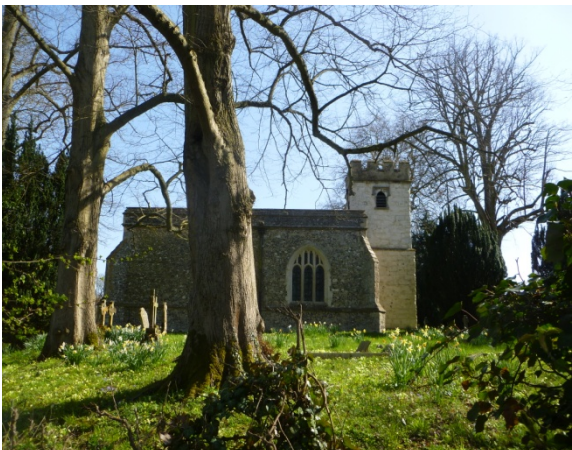
View of church from the north
