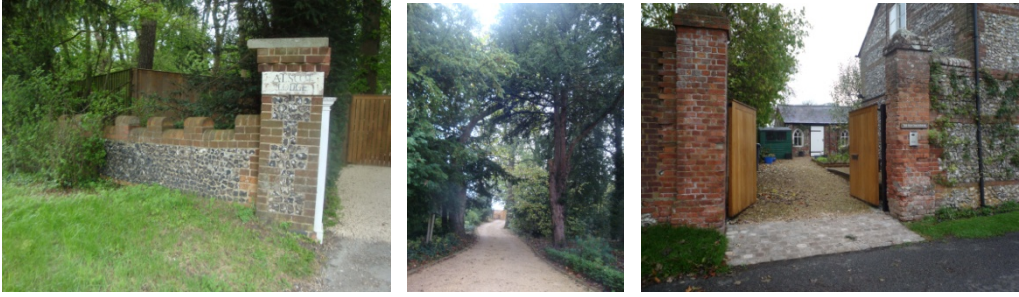
Main gateway off Longwick Road (left); drive (centre); stable yard gateway (right).
