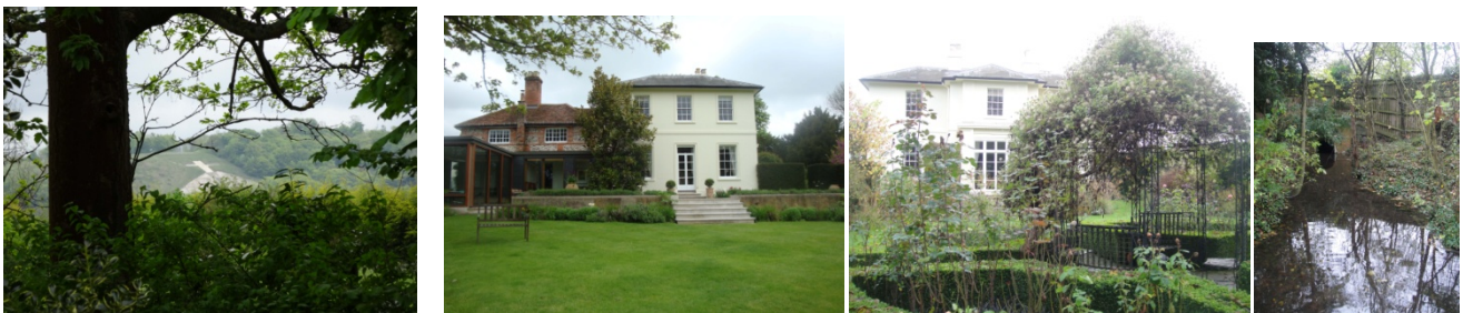
View from forecourt to Whiteleaf Cross (left); west, garden front and terrace (centre left); south, garden front (centre right); lake outlet below Longwick Road (right).
