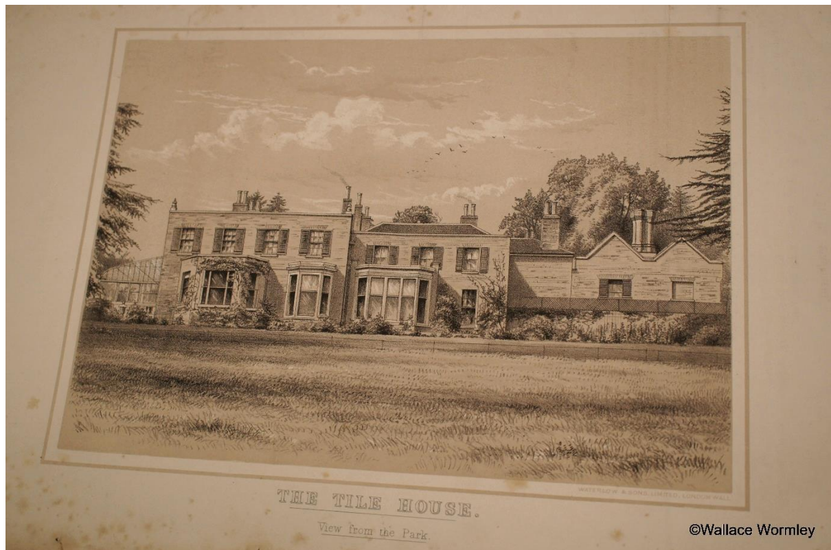
Front View of the Tile House, looking westward from the former Park, 1884 Auction Sale Particulars
