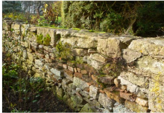
8. C20 retaining rubble wall
